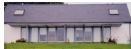
A long, modern window, broken up by vertical divisions to retain a vertical pattern.
