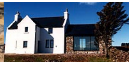
A modern extension using complementary and matching materials.
