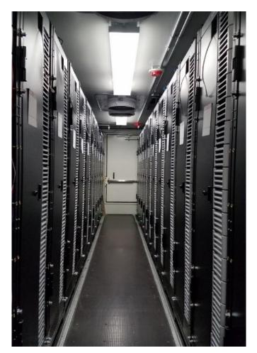
Note configuration of lithium ion banks, narrow access corridor and cooling vents fitted to ceiling.
