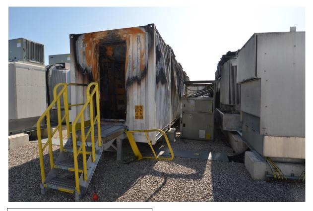
Image above: Exterior of unit with pressure damage to side.
