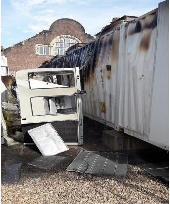
Image above: Taken from AIR Unit. Full extent of damage visible. Roof mounted cooling units ejected to side of unit. Pressure damage visible along length of unit. Note scorching of top edge of second unit to mid-right of image. Firefighting tactics mitigated further spread and damaged beyond original unit and blast.
