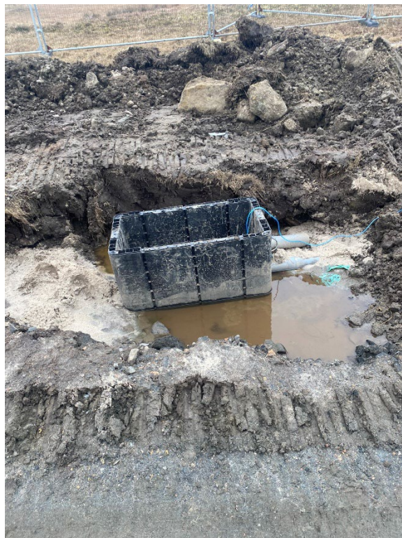
Photo 6 Installation of Openreach ducting and manholes
