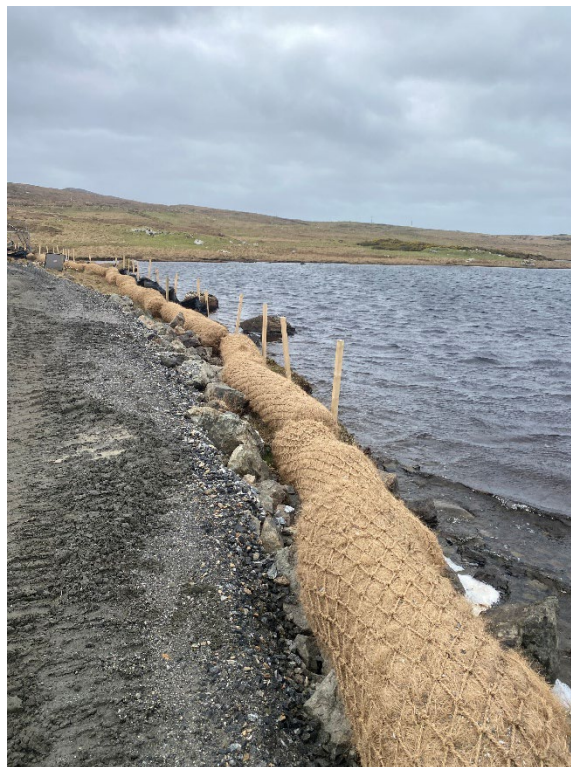
Photo 4 Silt mitigation measures
