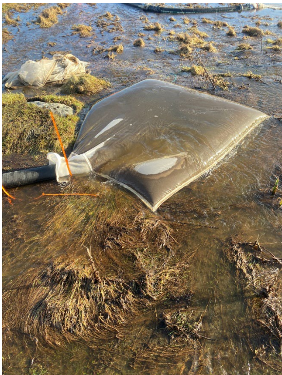
Photo 7 Silt bags to manage discharge from the desilters (removed from site within reporting period)
