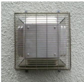
The outlet from the flue of the oil-fired appliance should be located externally at a safe distance from any opening, obstruction or combustible materials as follows:
